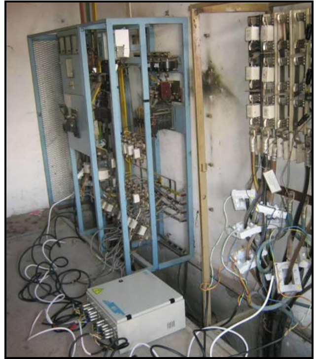
Figure 3. MIS-8 installed in TS 10/0.4 kV for closer localization of loss sources in the LV network
