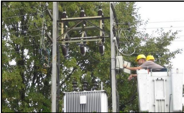
Figure 1. MIS-4S installed on pole TS 20/0.4 kV for checking the quality of power supply voltage
